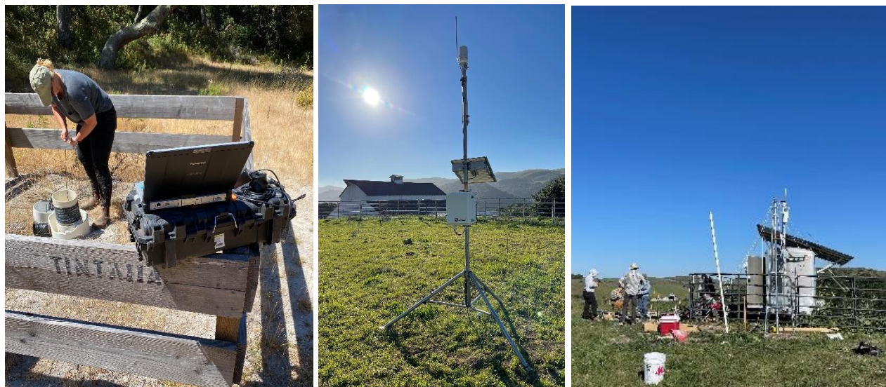
© Kelly Easterday/ TNC | From left to right: Installing a water level sensor; Weather Station at Jalama HQ; Installing the Motus tower at Bunker Hill.
